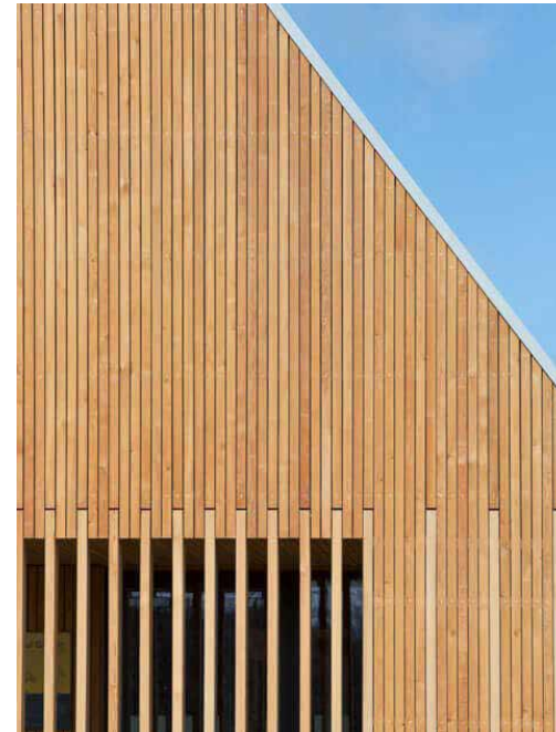
Building to be constructed using sustainable materials such as timber cladding
