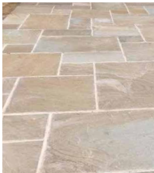
Sandstone paving to the plaza
